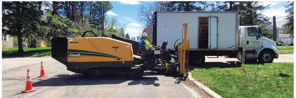
*An Arvig Drill Operator runs the directional boring machine that allows the installation of fiber optic cable underground.*
