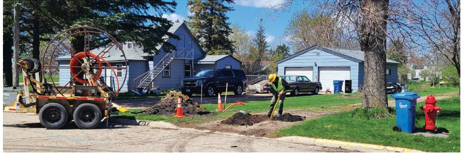
*This crew worker is looking for buried facilities by making a series of small test holes, called "potholing." This is a method to accurately locate the underground lines.*
