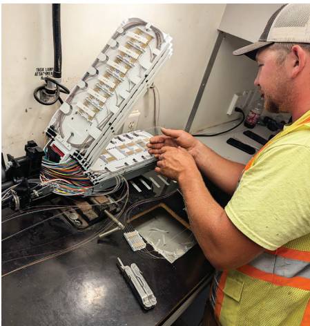
Braeden Long places repaired fiber lines housed within the BD7 fiber pedestals which are typically found in road right-of-ways on mile section lines.
